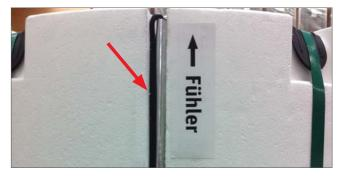
**5)** Later on, when the sensor needs replacing after several years, for instance, this can be done via the lid. To do this, you only need to remove the lid and not any of the other insulating shells; see the marking on the picture.
